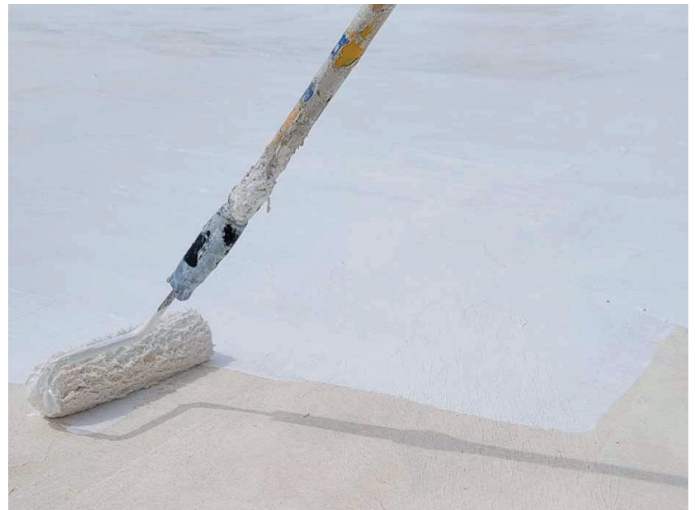
APPLICATION OF 3 COATS OF ELASTOMERIC COATING
