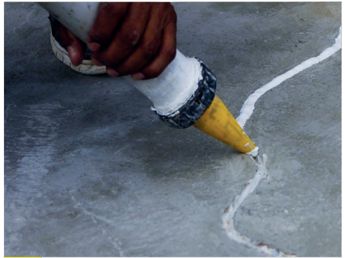
CRACK FILLING WITH ZK-007 PLASTICIZED CHEMICAL
